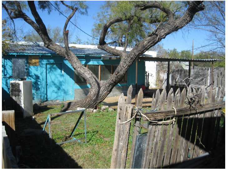
Existing patio area behind building
