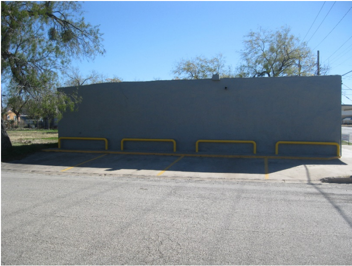
Looking south at building (1218 MLK)
