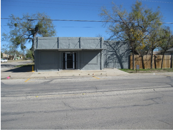
Looking east at Building (1218 MLK Dr.)
