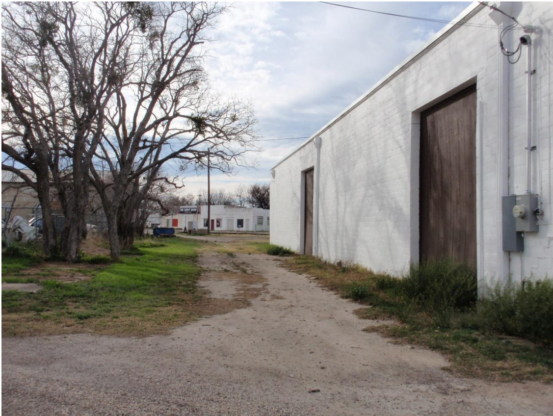
East-West alley adjacent to 805 South Chadbourne Street
