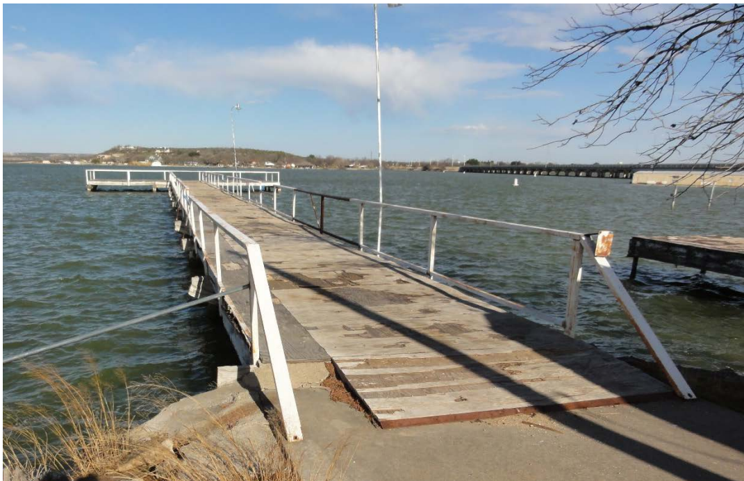
Figure 1: Overview of Pier Viewed from the Abutment
