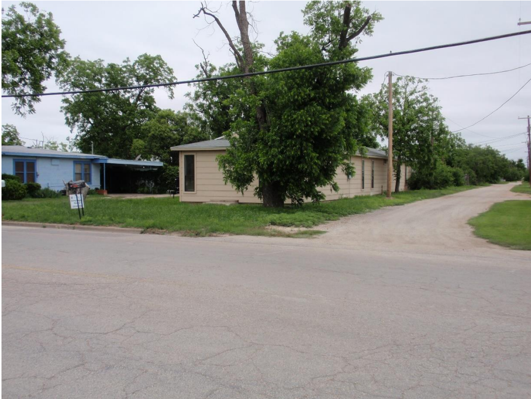
South Alley Side of Subject Property
