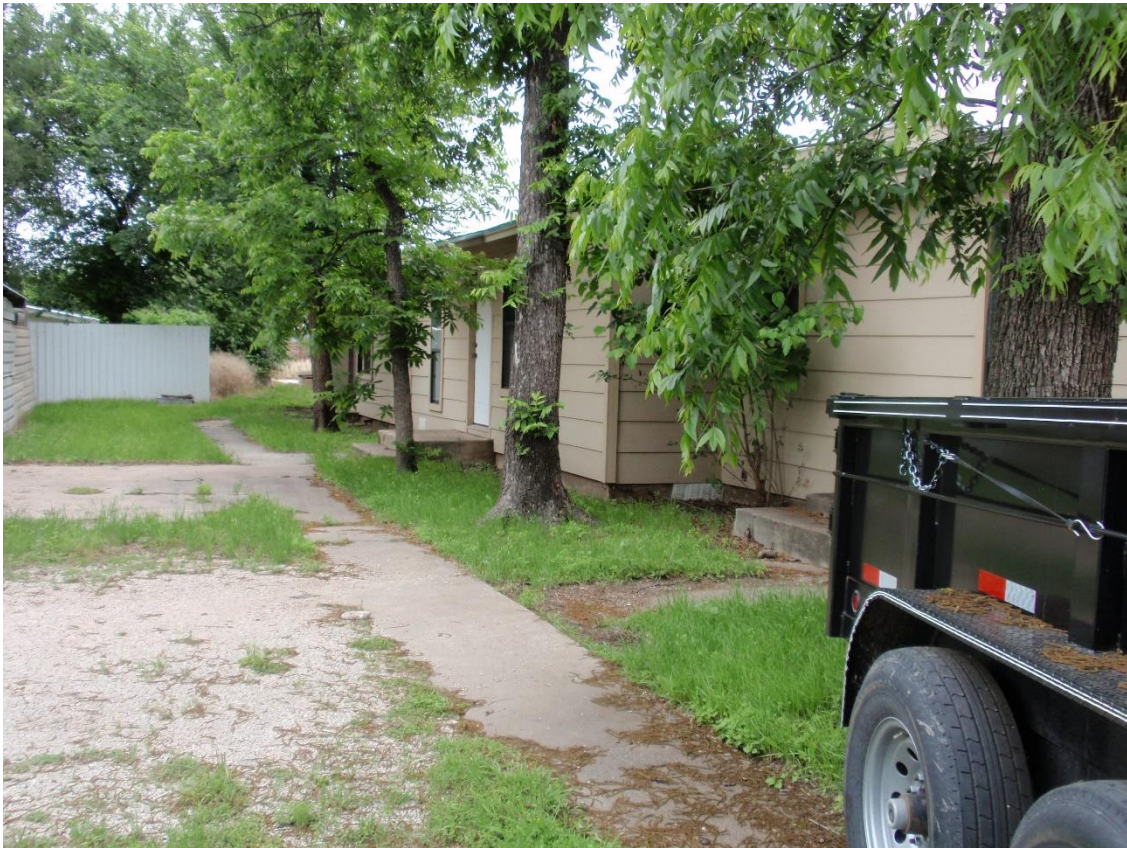
Northern side of the existing structure
