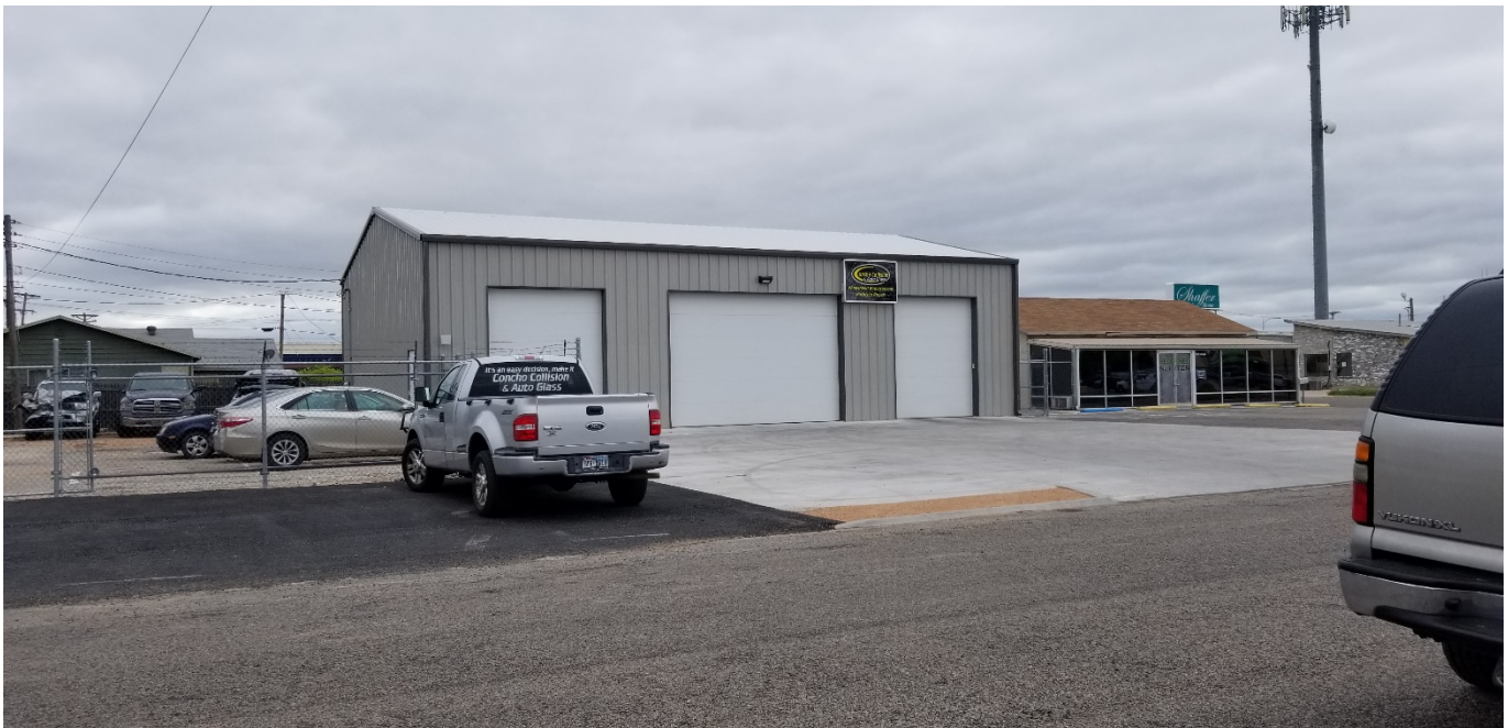
STRUCTURE OFF TYLER
