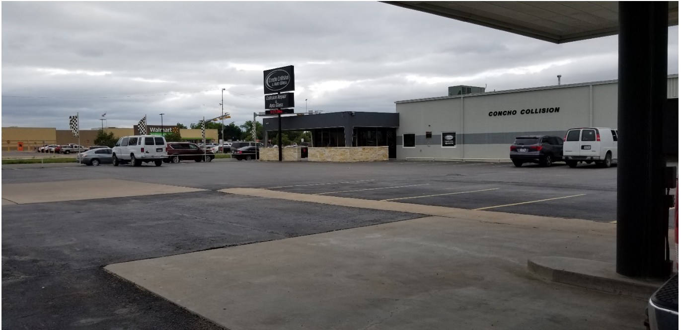
MAIN STRUCTURE AND OFFICE
