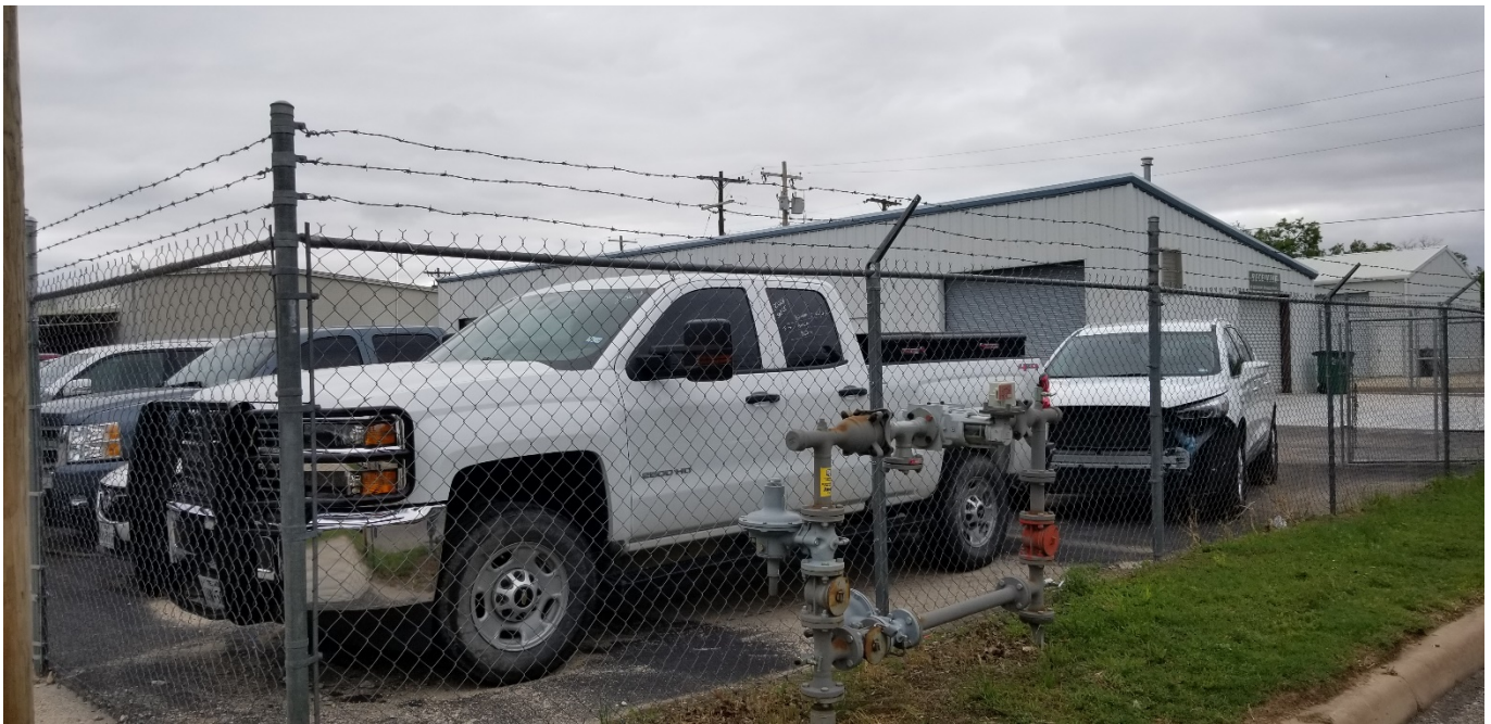
CLOSEUP OF EXISTING FENCING ALONG HARRISON AND COLORADO
