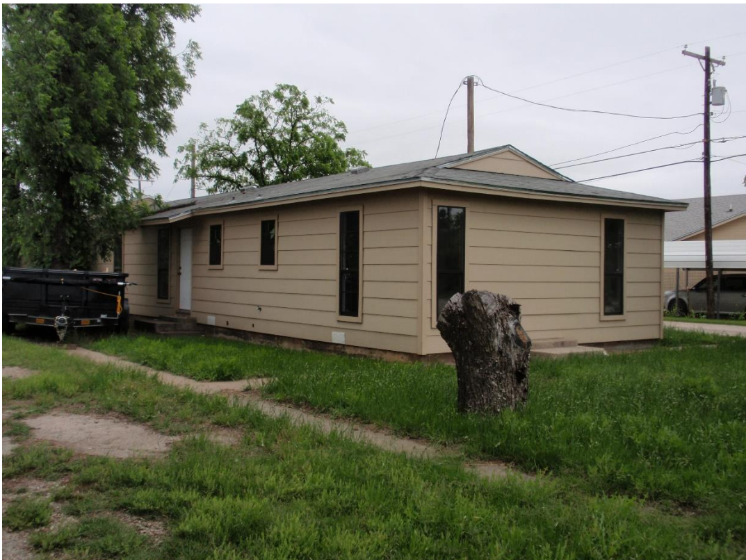
Northeast Corner of the existing structure
