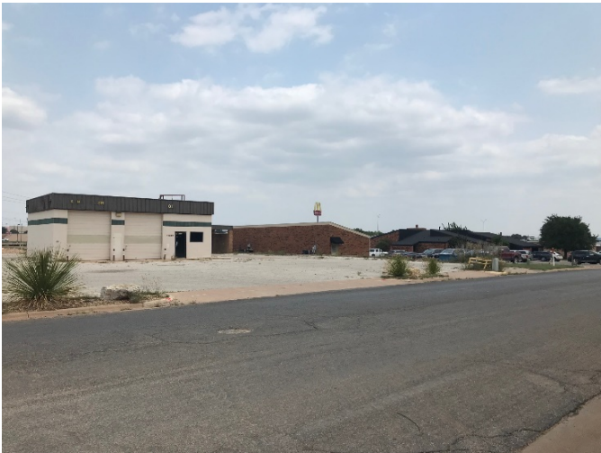
IMMEDIATELY EAST AT FUTURE OFFICE/SHOP
