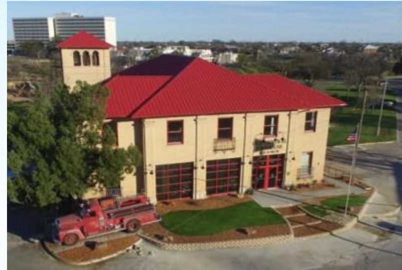
Façade with firehouse doors 1 st floor: Brew - Coffee/Beer/Wine gathering area 2 nd floor: Bed & Breakfast (4 room area) Quasi-museum with fire house artifacts
