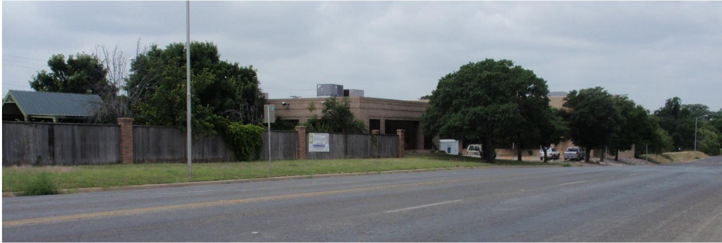
Existing School and Office Building south of West Harris Ave.
