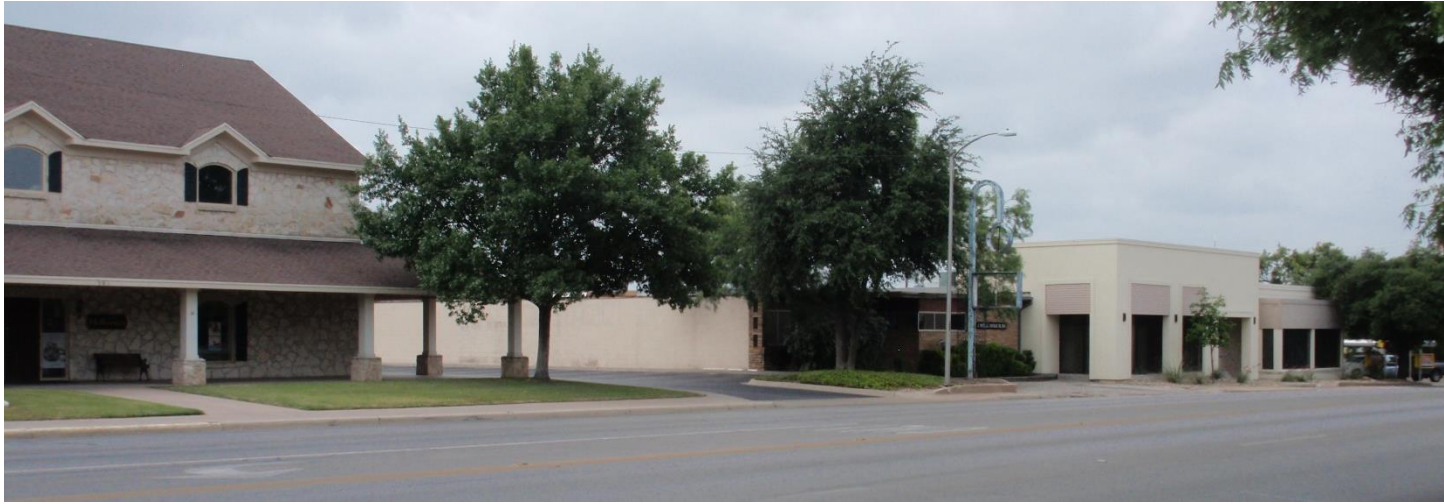
Existing Office and Retail south of West Beauregard Ave.
