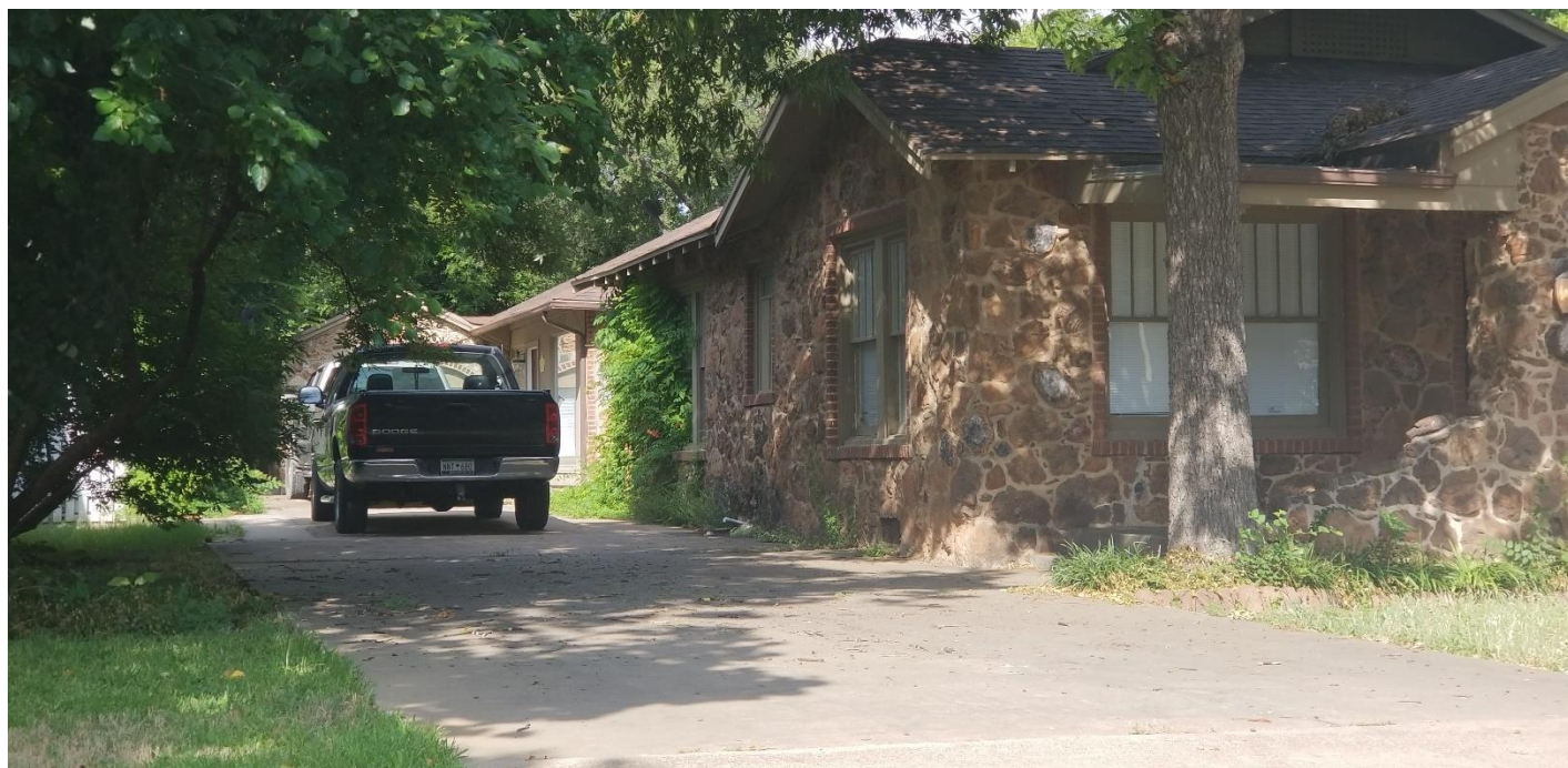
Close up of the back apartment
