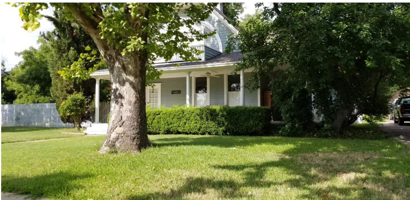
House at 219 S Washington
