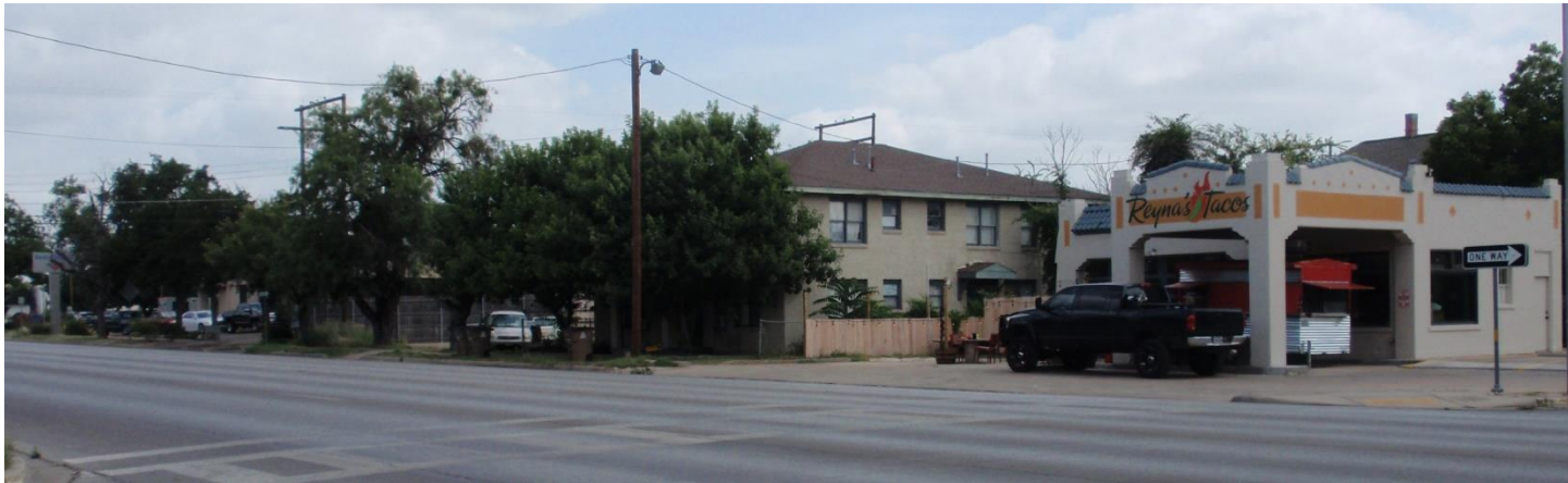
Existing Retail and Multi-family at corner of West Concho Ave. & South Abe St.
