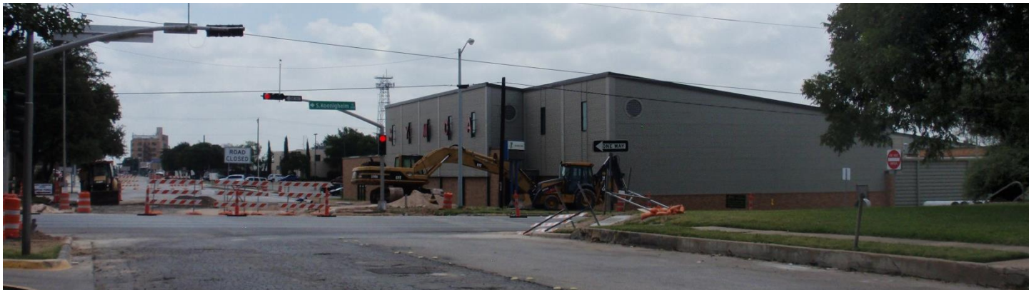
Existing YMCA at the corner of West Concho Ave. and South Koenigheim St.
