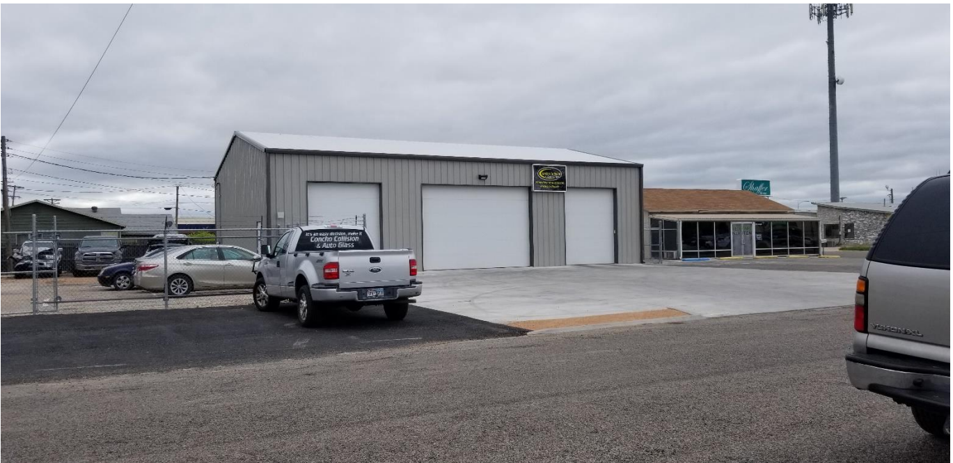
STRUCTURE OFF TYLER
