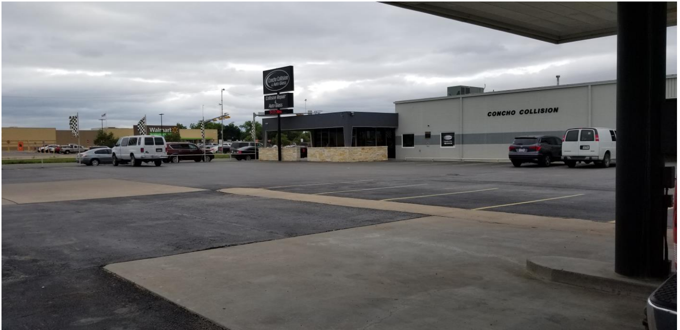
MAIN STRUCTURE AND OFFICE
