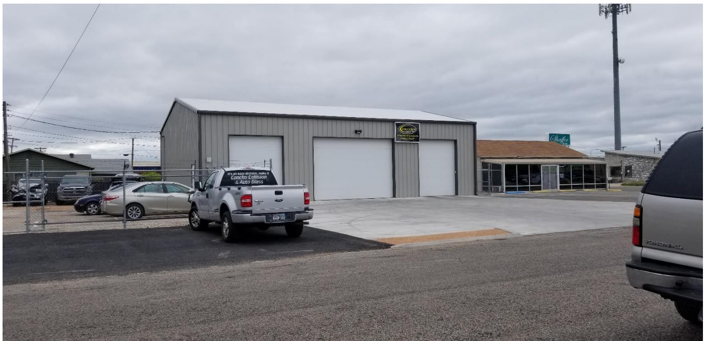
STRUCTURE OFF TYLER
