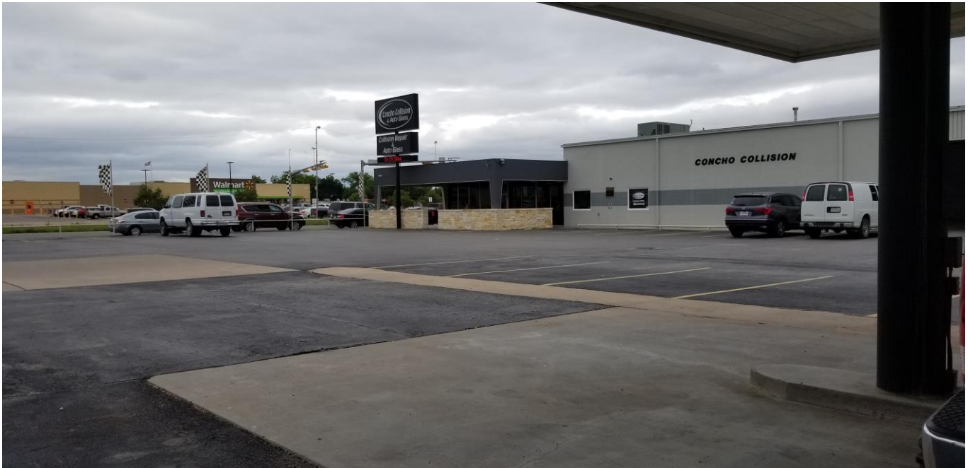
MAIN STRUCTURE AND OFFICE
