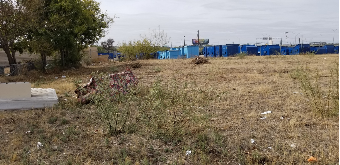
Archer St. at alley with electric pole removed
