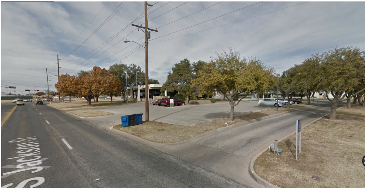
SIDE IMAGERY OF THE SUBJECT PROPERTY (South Jackson Frontage)
