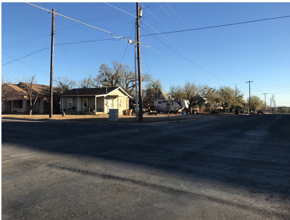
Residence east of the subject property
