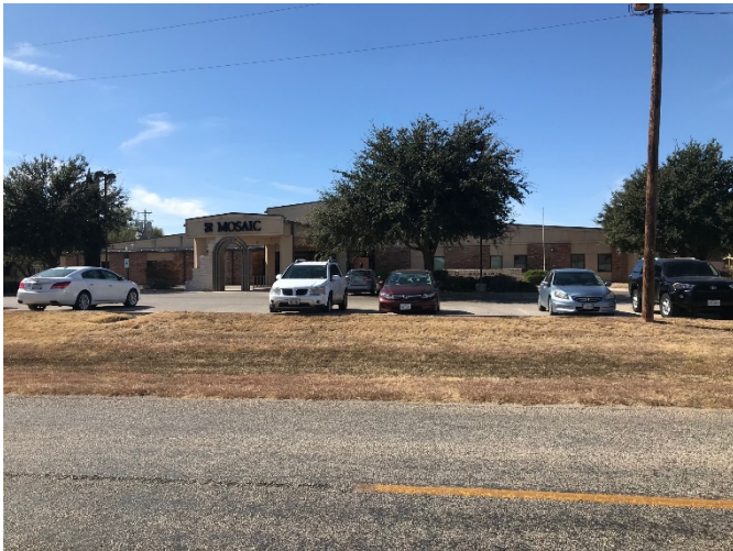
WEST AT MOSAIC PROPERTY
