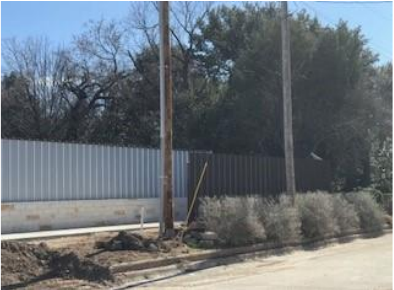
Photo of subject fence
