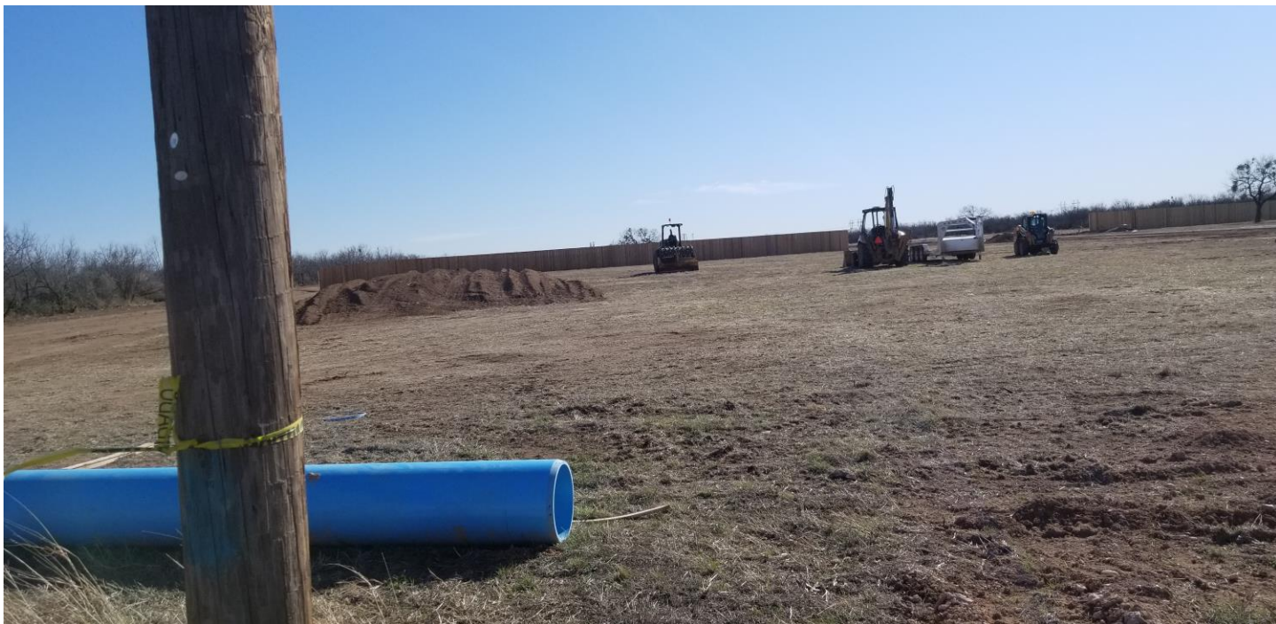
Subdivision work in progress
