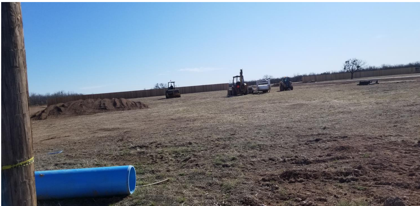
Old Stone Rd. being constructed. Note the separation fence between commercial and residential.
