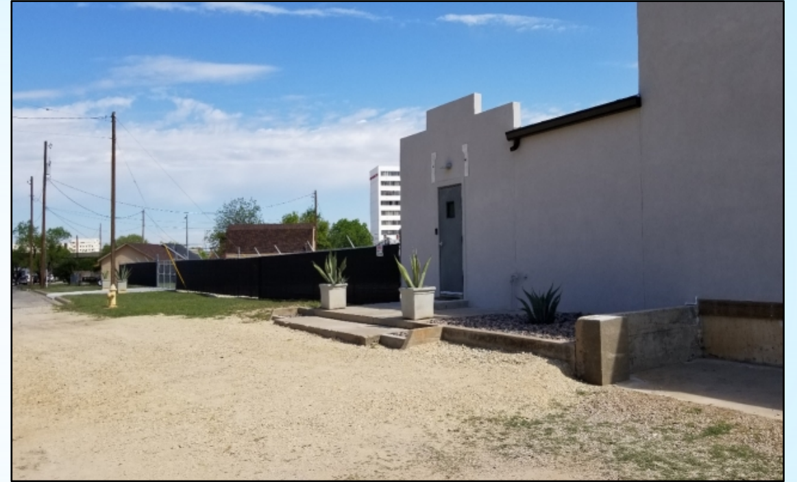
Remodeled office and storage building
