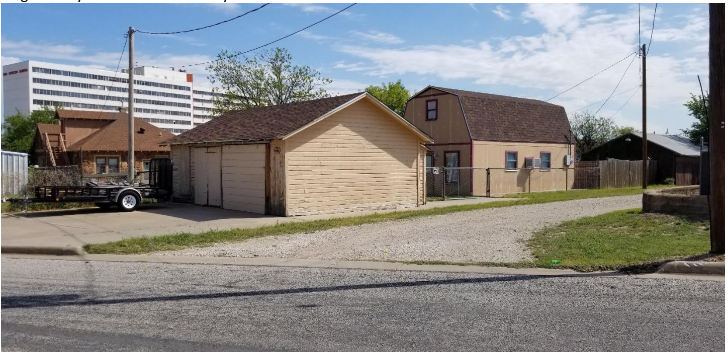
Single family home across the alley
