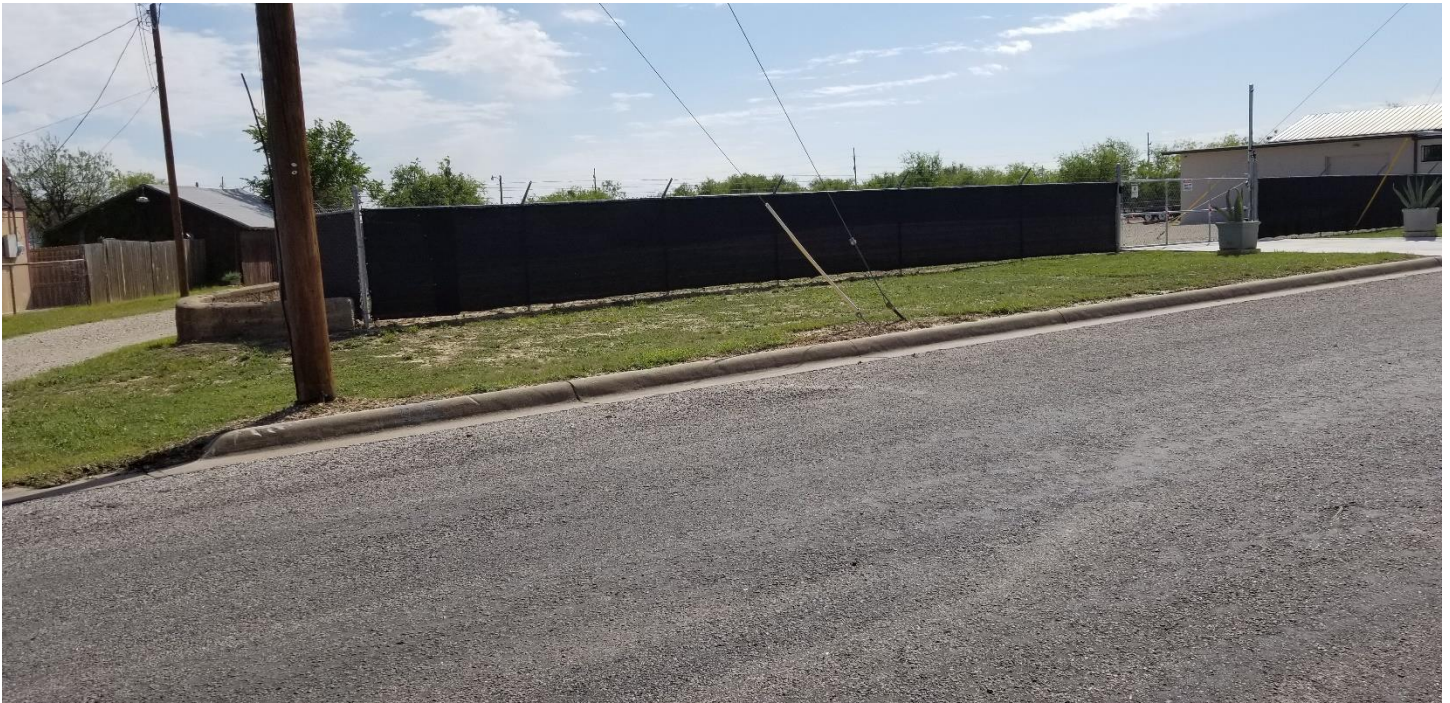
Site showing fence and exterior of the property
