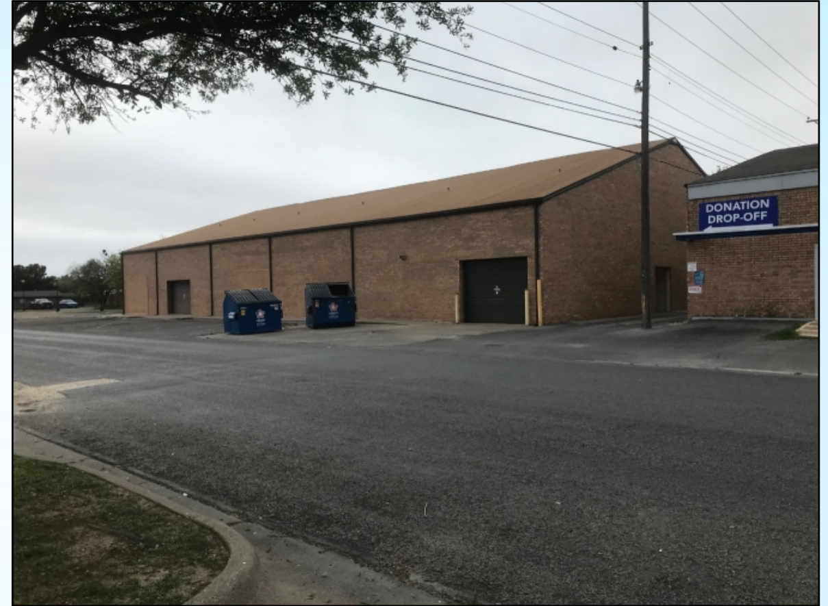
West at 2302 W. Harris Ave. (CP20-03)
