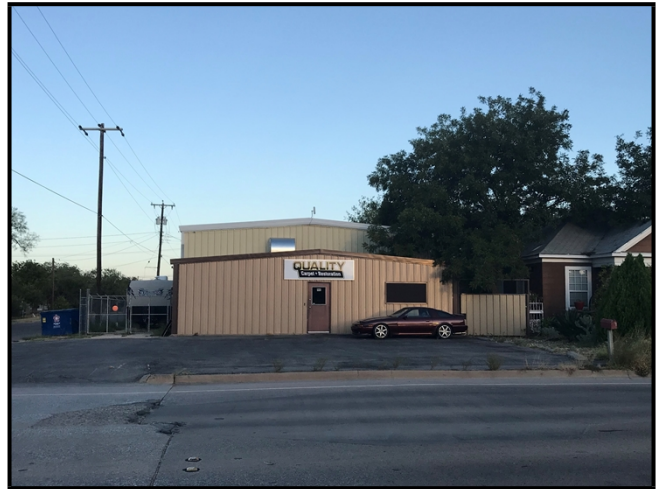
Commercial south of subject property
