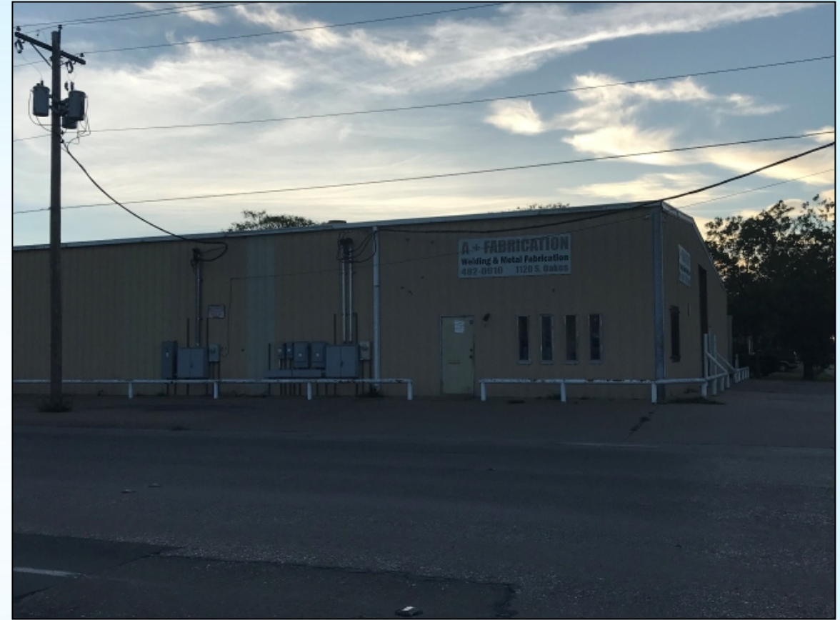
Commercial across S Oakes Street
