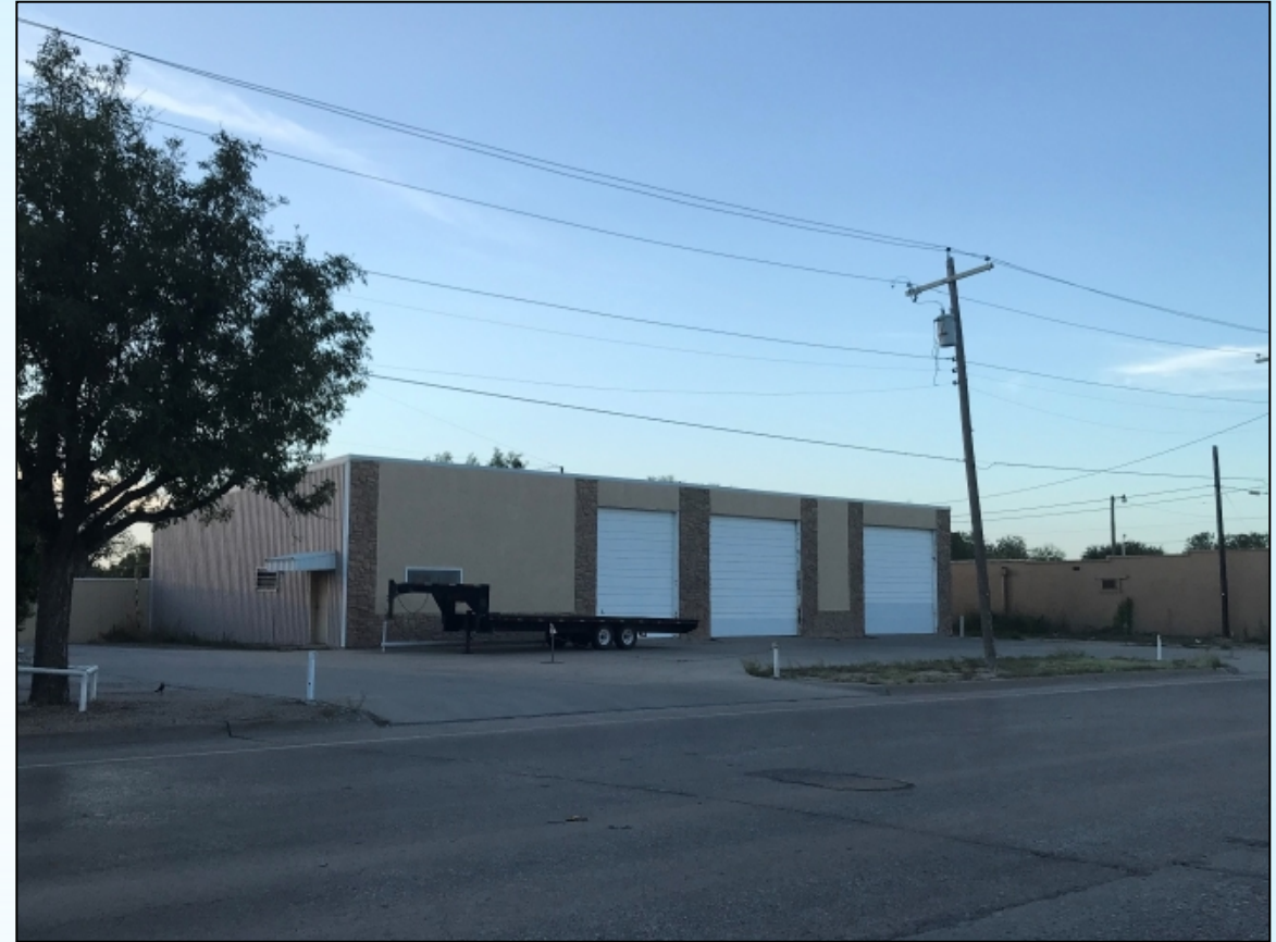
Commercial across S Oakes Street
