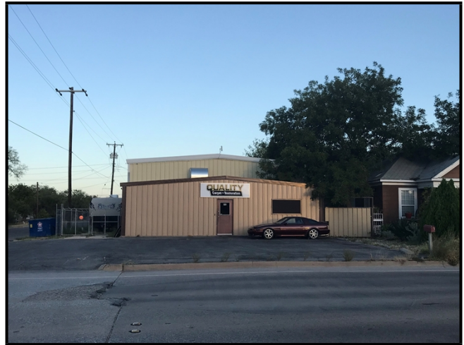
Commercial south of subject property
