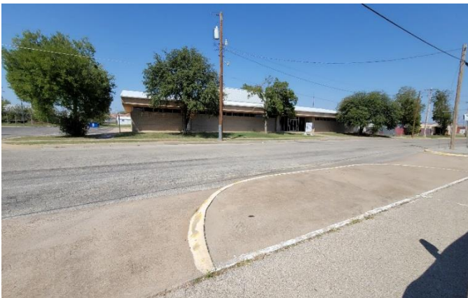
Old Emergency Shelter building
