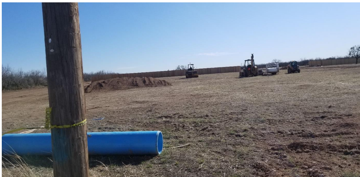
Area to the south of existing development road area to AEP easement
