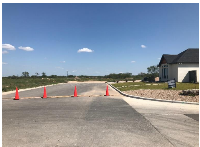
NORTH ON ENCLAVE COURT AT LINVILLE LN
