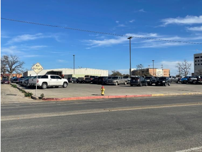
EXISTING MAINTENANCE FACILITY (WOODROW ST)
