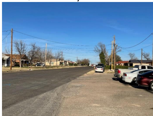
WEST 23 RD ST. LOOKING EAST ( FUTURE ABANDONMENT AREA )
