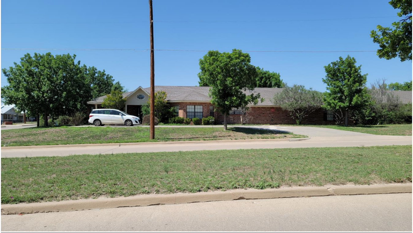
Residential facility at 404 Preusser Street
