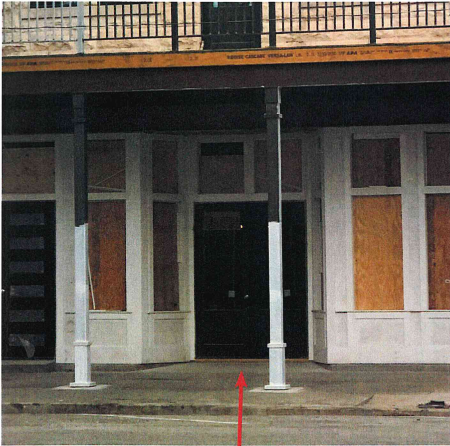
tile installation location
