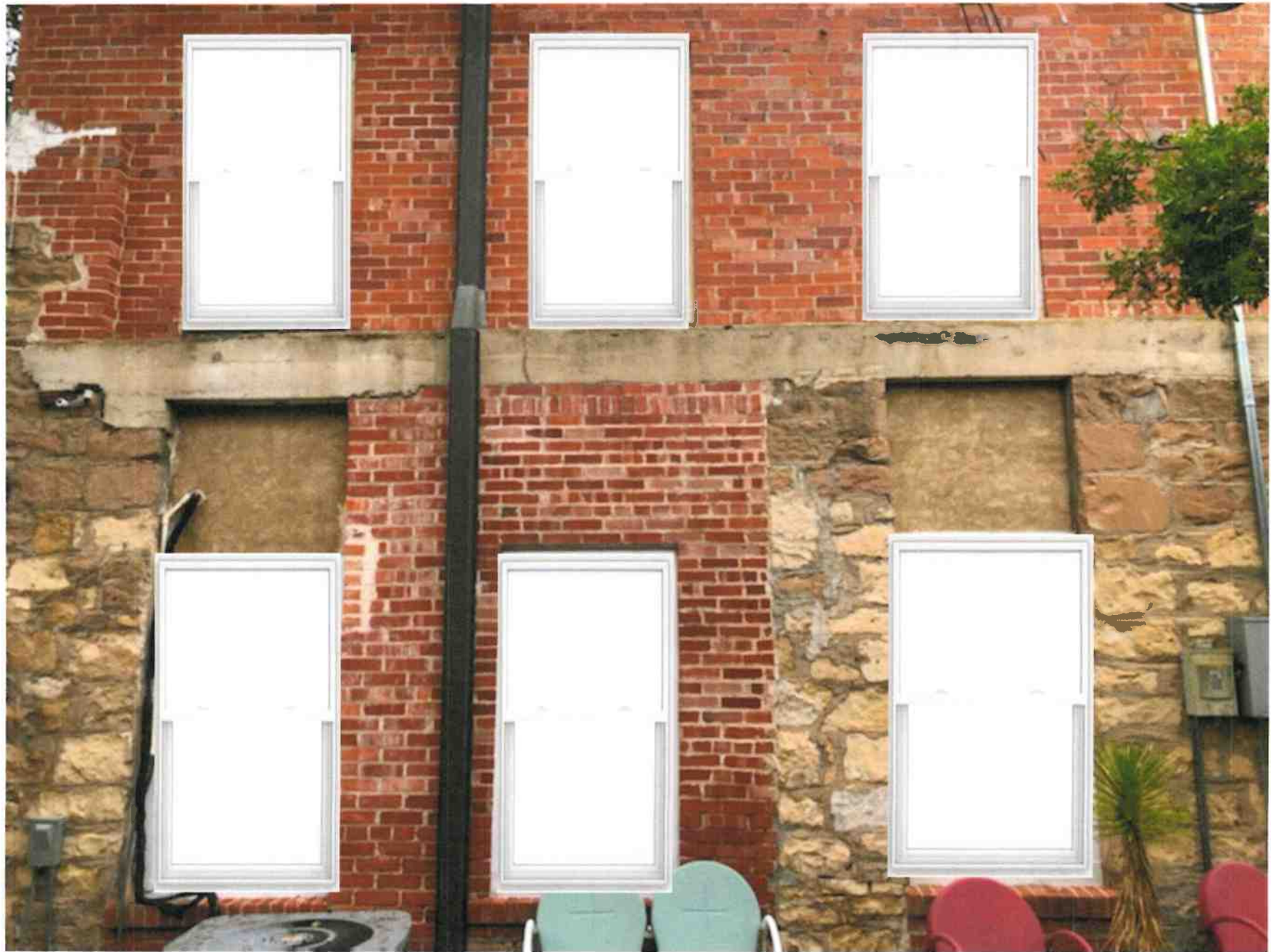
new windows installed
