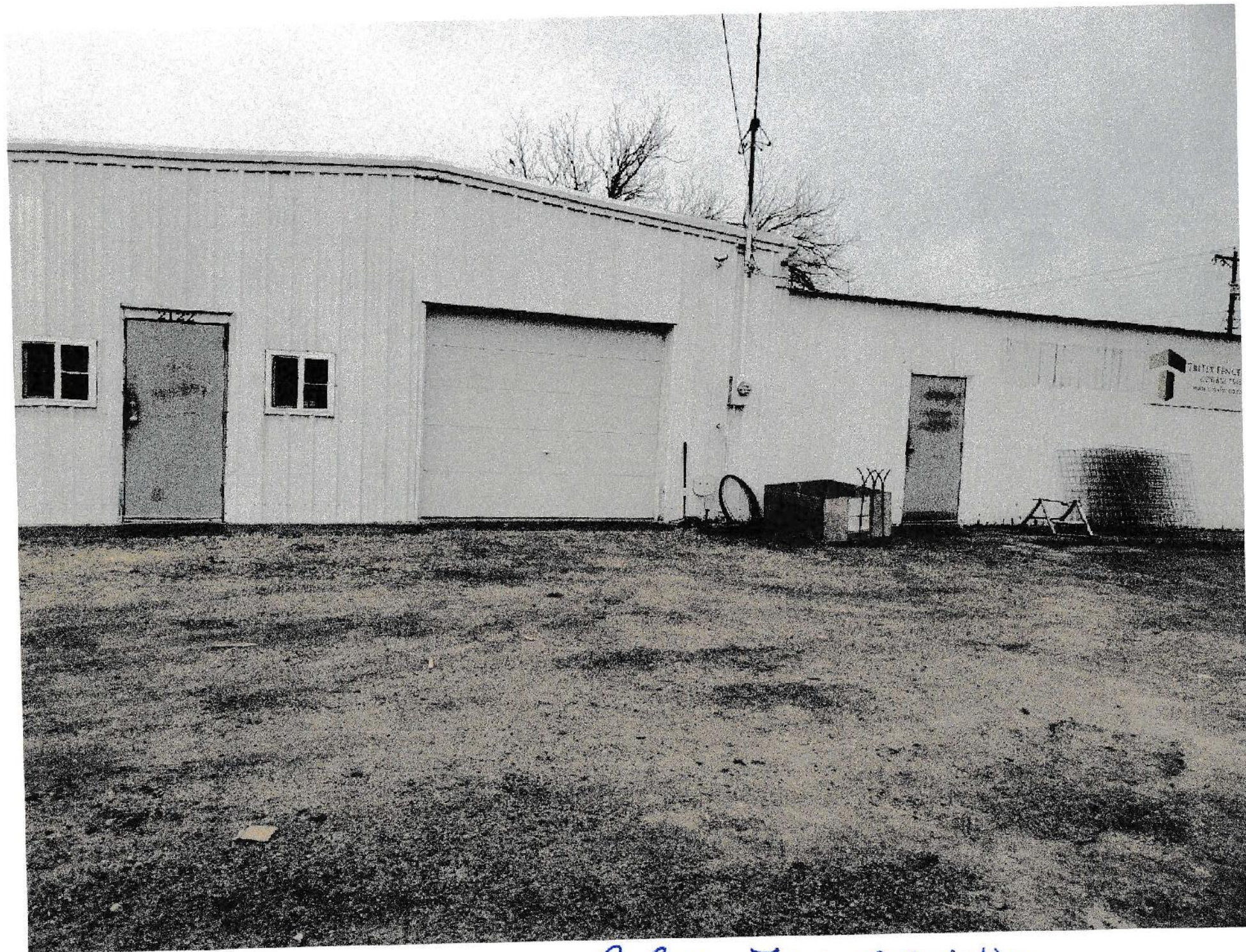
Before - Front of Building
