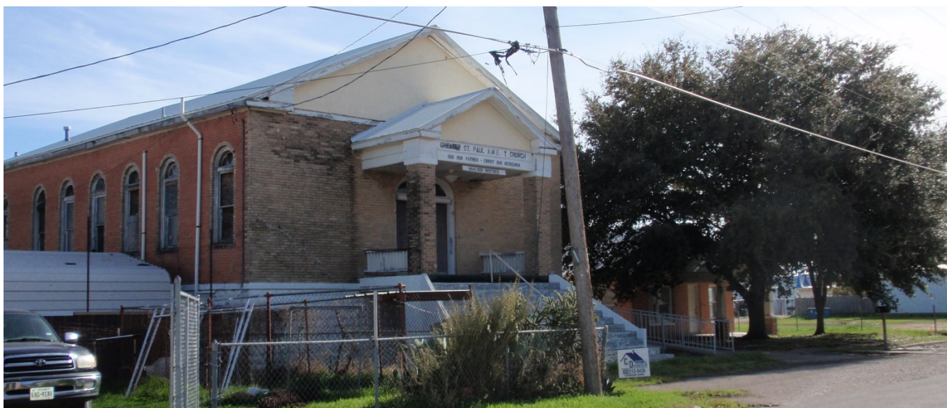
Existing church building W 3 rd St.
