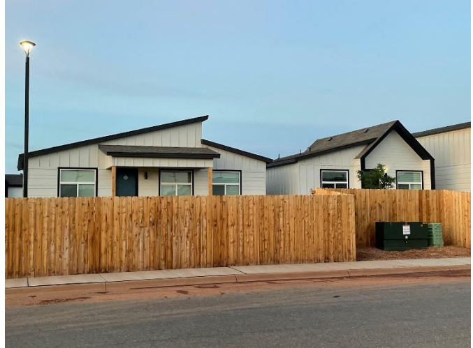
EXISTING UTILITY BOX – RECOMMEND MOVE BACK FRONT FENCE TO MATCH JOG LINE
