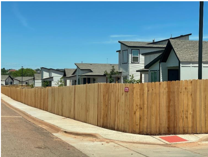
MIDDLE VIEW OF FRONT FENCE
