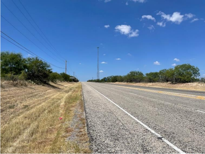
NORTHBOUND ON ARDEN RD.
