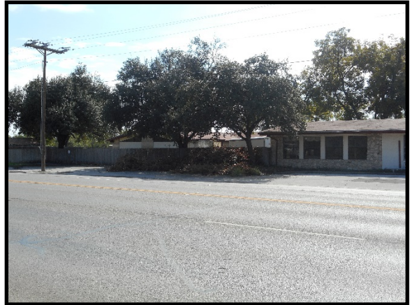
Southeast at Property
