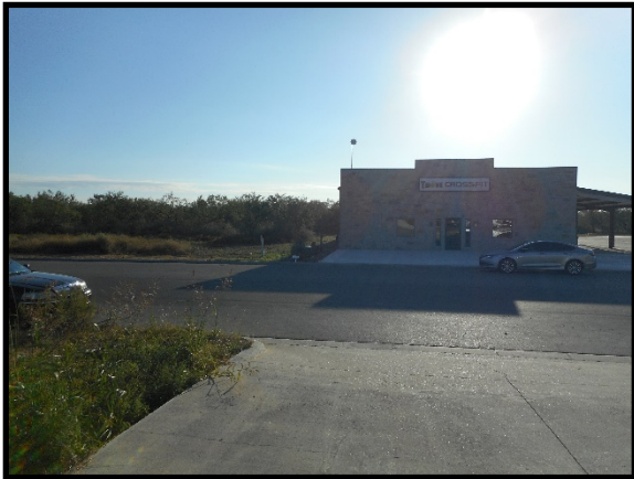
West (existing Crossfit Gym)
