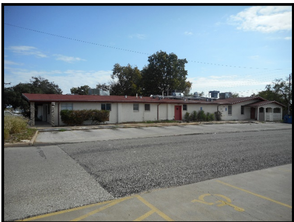
West elevation looking at building
