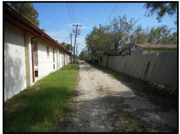
Rear of Building (South)
