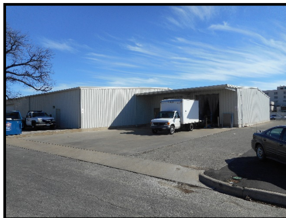
Shannon Storage Facility (115 Woodrow St.)
