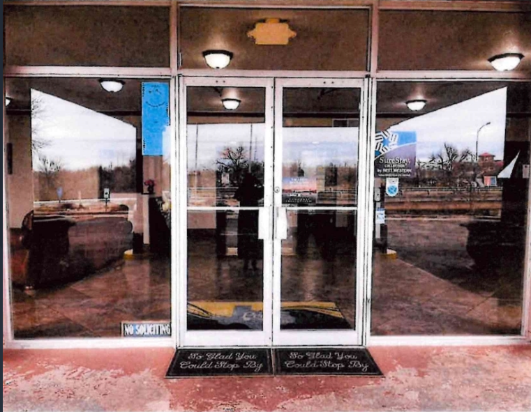
Existing Main Lobby Doors
