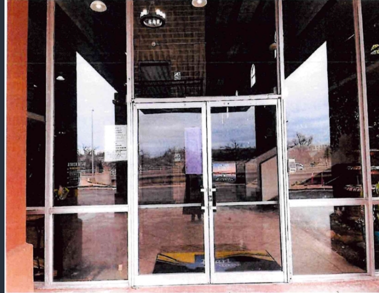
Existing Side Lobby Doors
