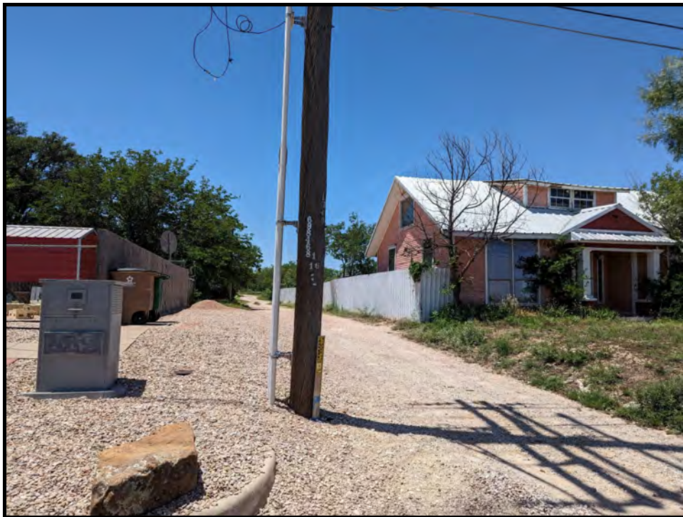
Taken from Rust St looking west at the alley that is the primary access to this lot.
