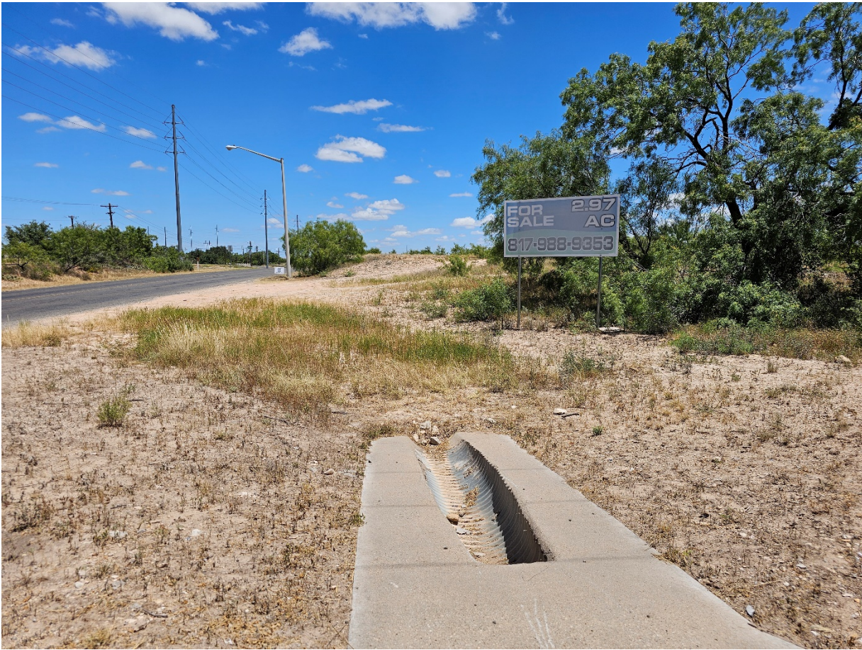
Entrance off of The Crossings site where the Attorney General's Building is located. It shows the existing drainage structure carrying water from across The Crossings state property to this site where it naturally flowed.
