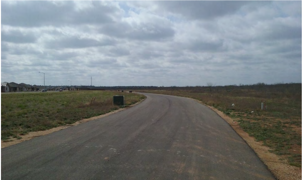
LOOKING SOUTH FROM WILLKE DRIVE
