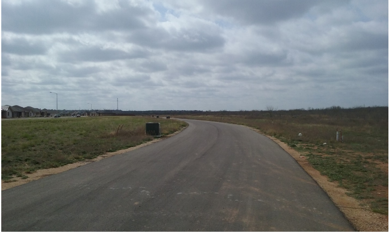
LOOKING SOUTH FROM WILLKE DRIVE
