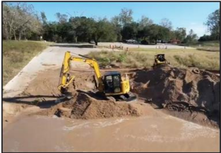
Figure 1: Dredging Project in Progress
