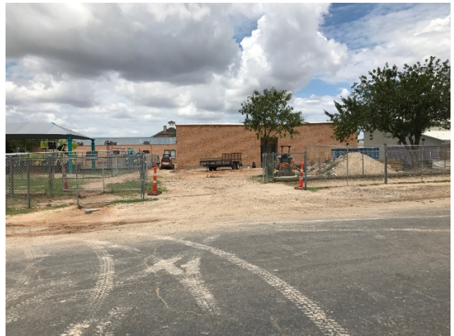
PORTION OF FENCE FACING E. HIGHLAND BLVD. (TEMPORARILY REMOVED)
