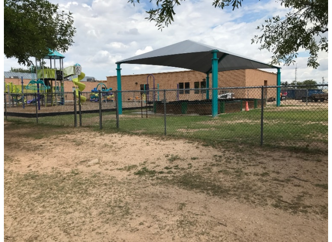
FENCE FACING BURGESS STREET (ON PRIVATE PROPERTY)
