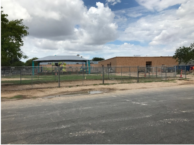
FENCE FACING EAST HIGHLAND BLVD. (REQUIRES ENCROACHMENT APPROVAL)
