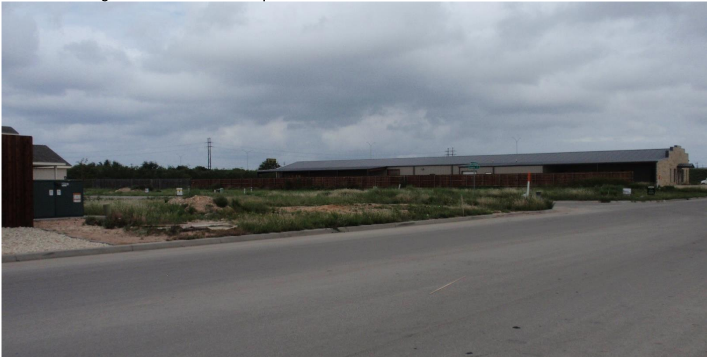
Looking North toward the Properties on Colonial Drive from North Bentwood Drive
