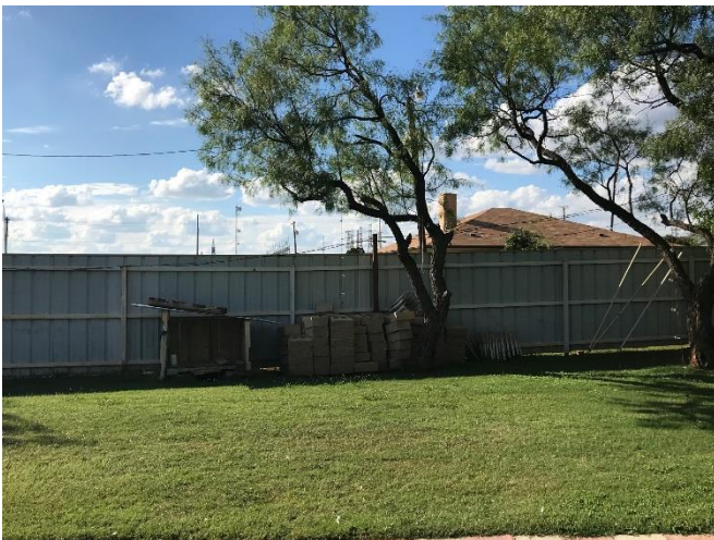
EXISTING PRIVACY FENCE (WEST)
