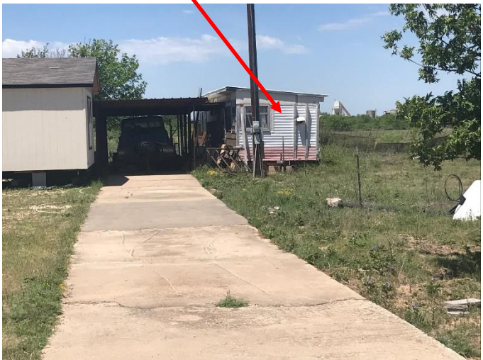
EXISTING MOBILE HOME (TO BE REMOVED)
