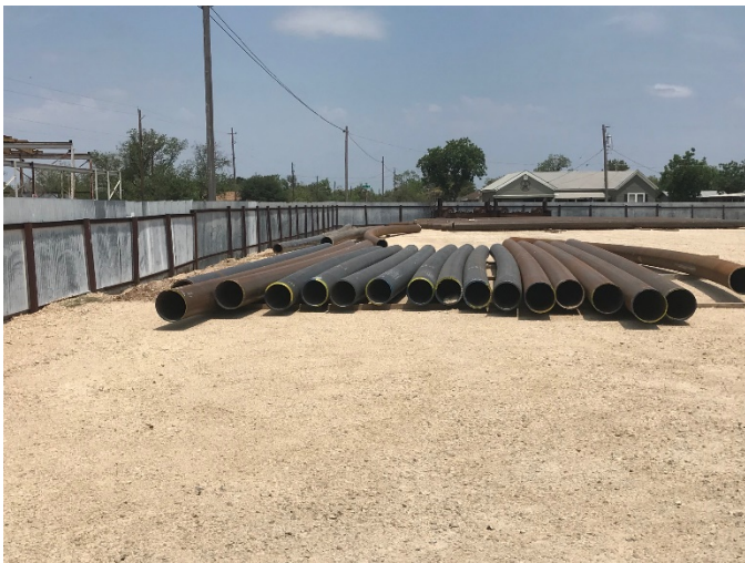
INSIDE PROPERTY LOOKING NORTH
