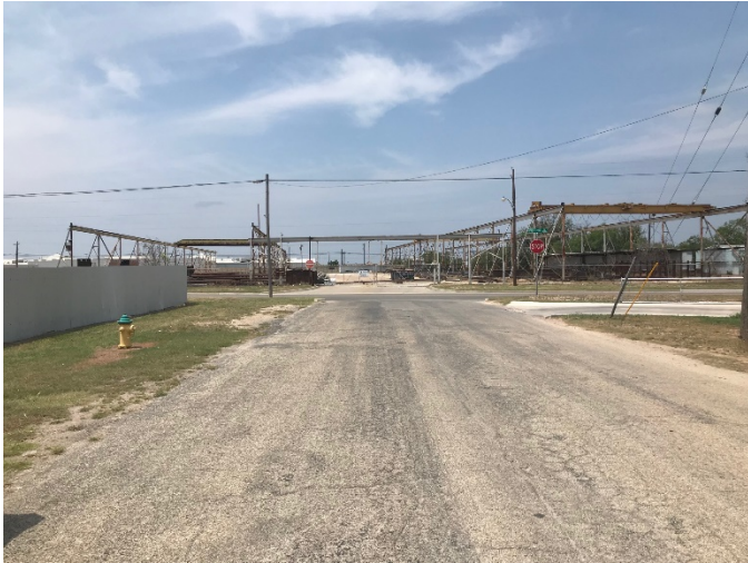
LOOKING WEST AT GRAPE CREEK ROAD
