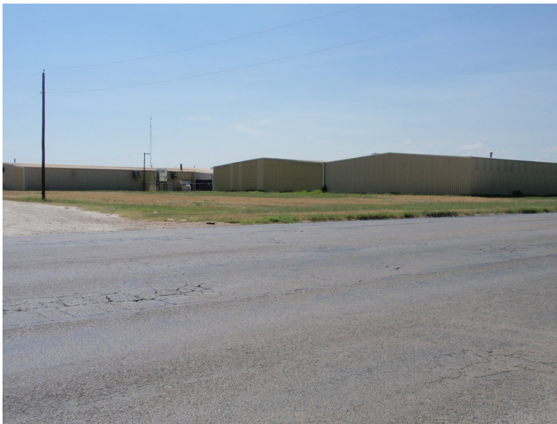
Property Directly Southeast across South Bell Street
