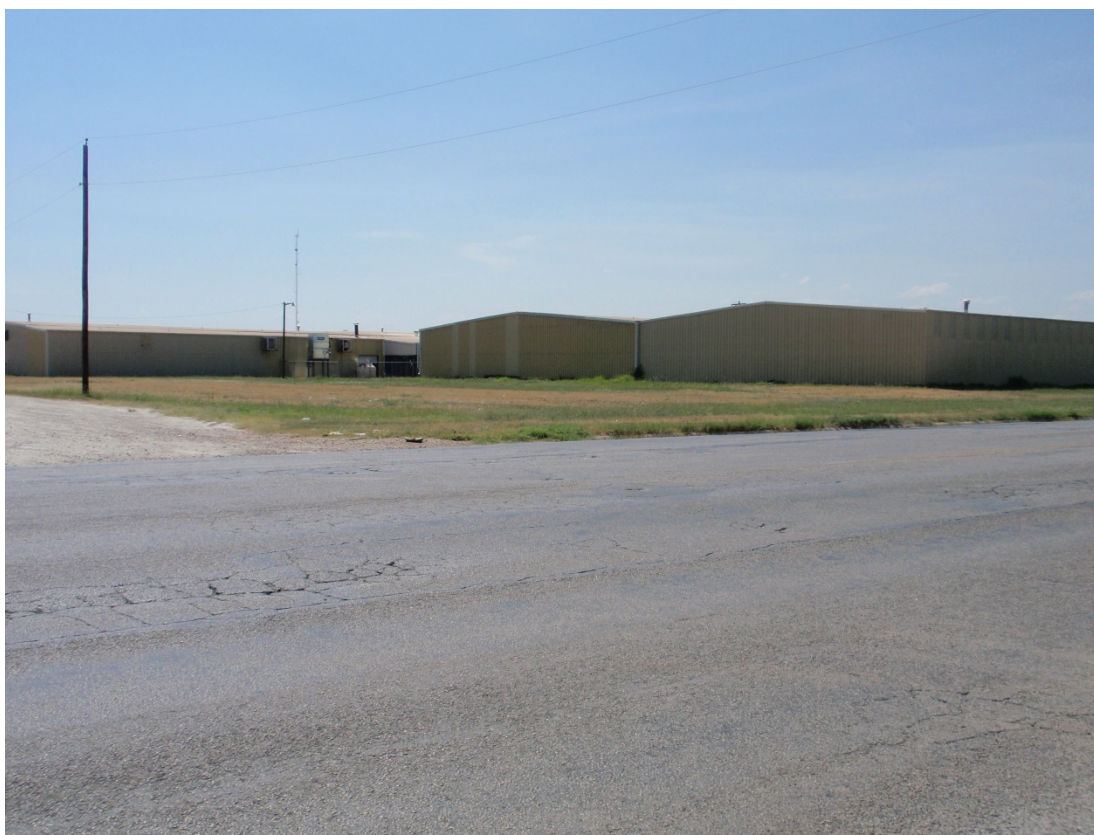
Property Directly Southeast across South Bell Street
