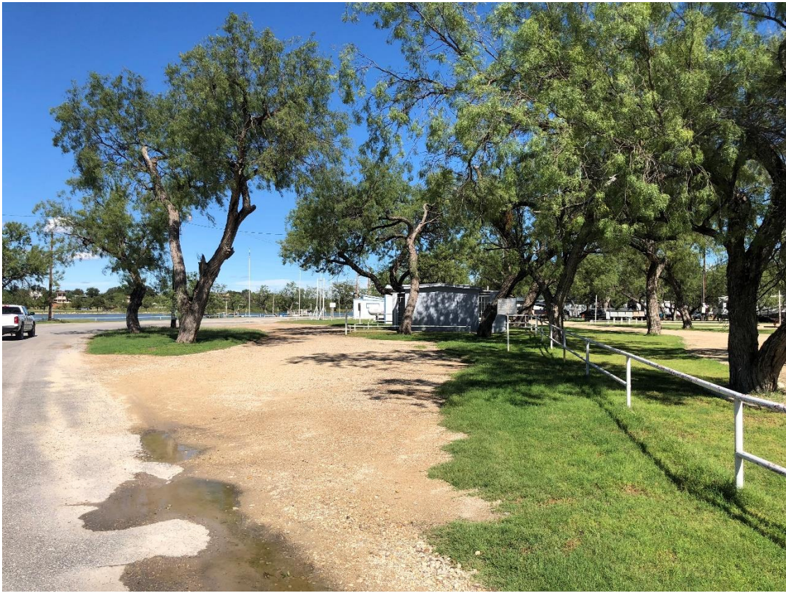
Park Restroom Facility
