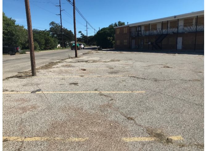
EXISTING PARKING AREA
