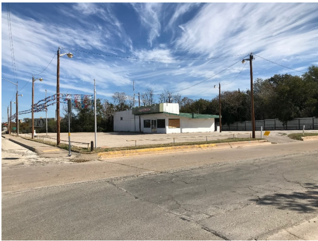
SOUTHEAST AT PROPERTY
