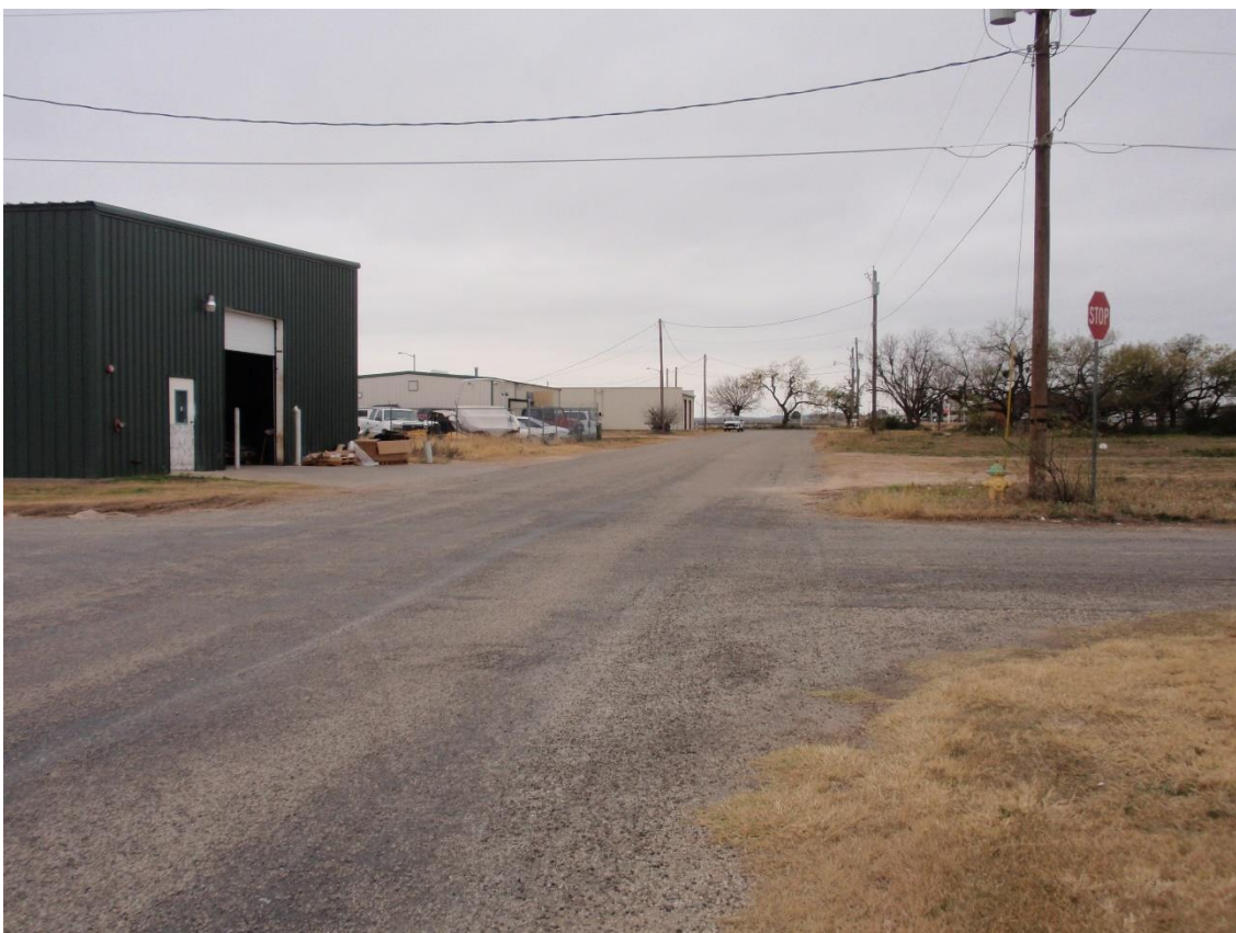
Commercial Properties South of Subject Property
