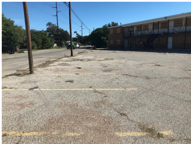
EXISTING PARKING AREA
