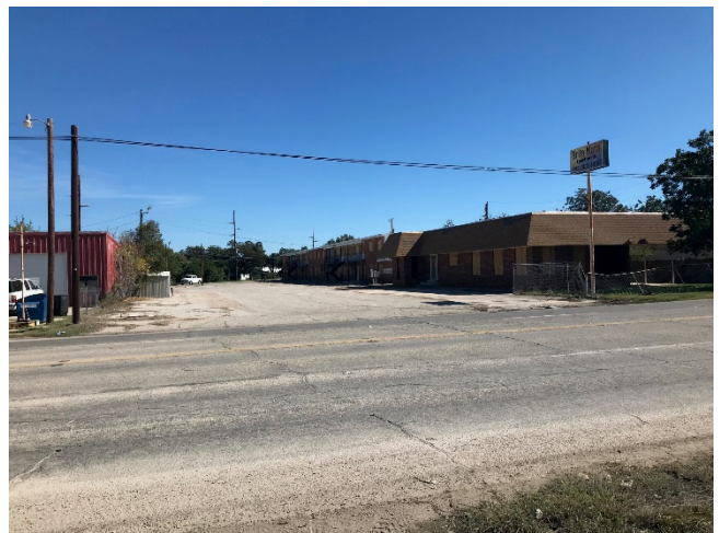
EAST LOOKING AT PROPERTY
