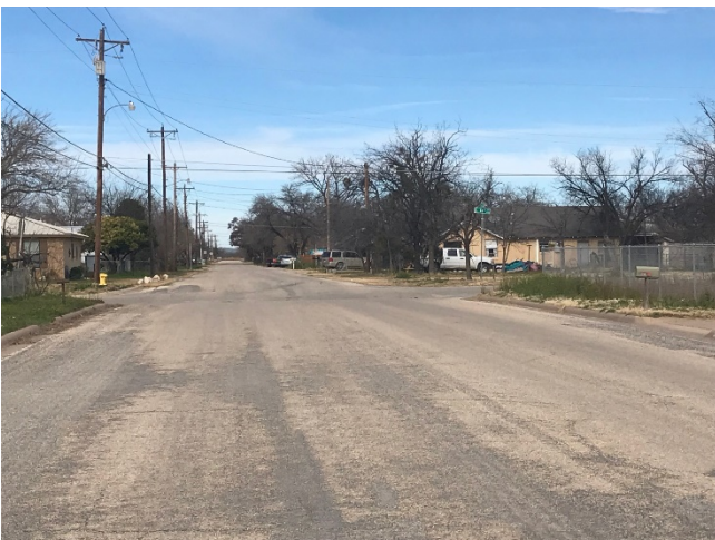
LOOKING NORTH ON BOWIE ST
