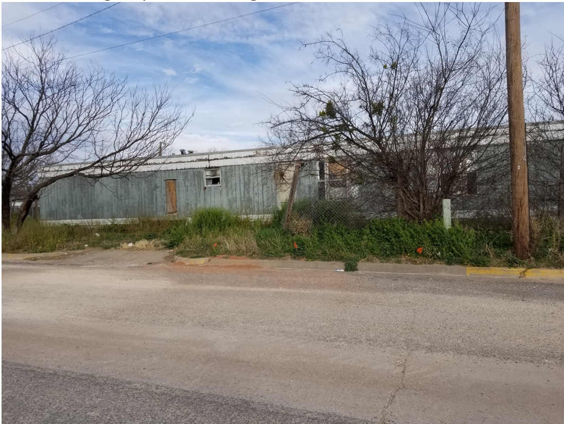
Looking east across Lowrie Ave.
